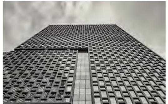
The external cladding characterises the structure through the harmonious interweaving of two materials: the glass, totally transparent, and the Laminam slab, completely opaque, chosen here in the Calce series, in the colour Nero. The lightness of the large surfaces of the 1000x3000mm size, 3mm thick, reinforced on the back with fibreglass, also guarantees extreme durability through excellent weather and wear resistance.
